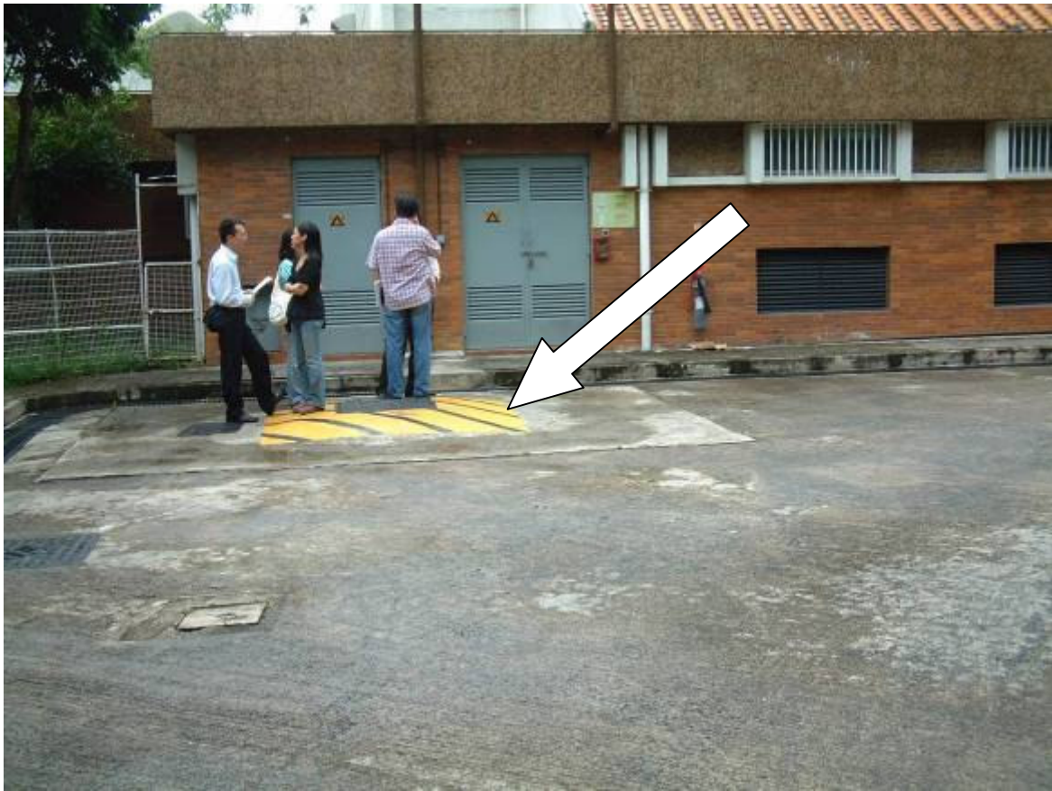
Photo 7 – Underground Fuel Tank in Coffin Crematorium
