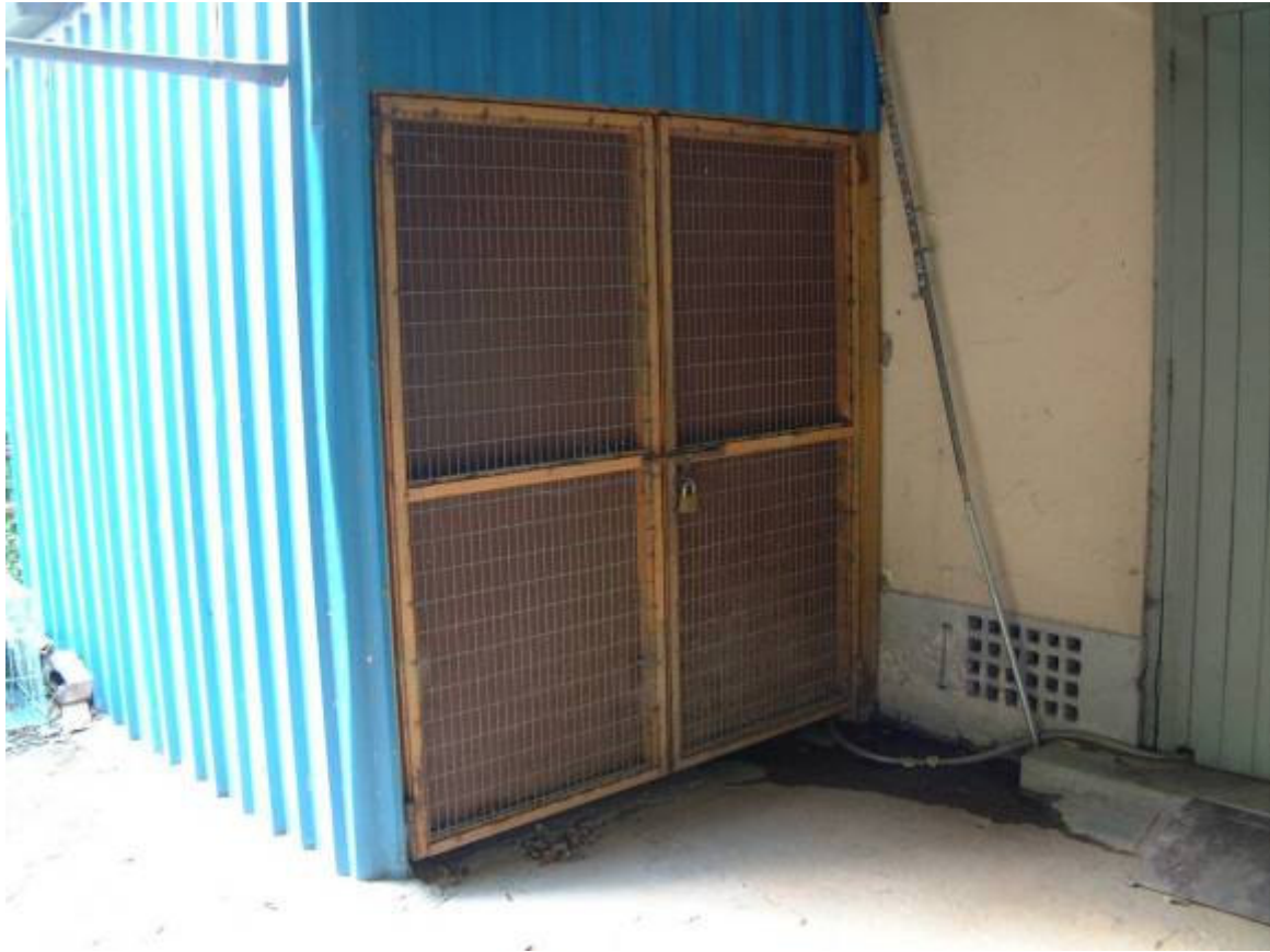
Photo 17 – Dangerous Goods Store in Skeletal Cremator Building
