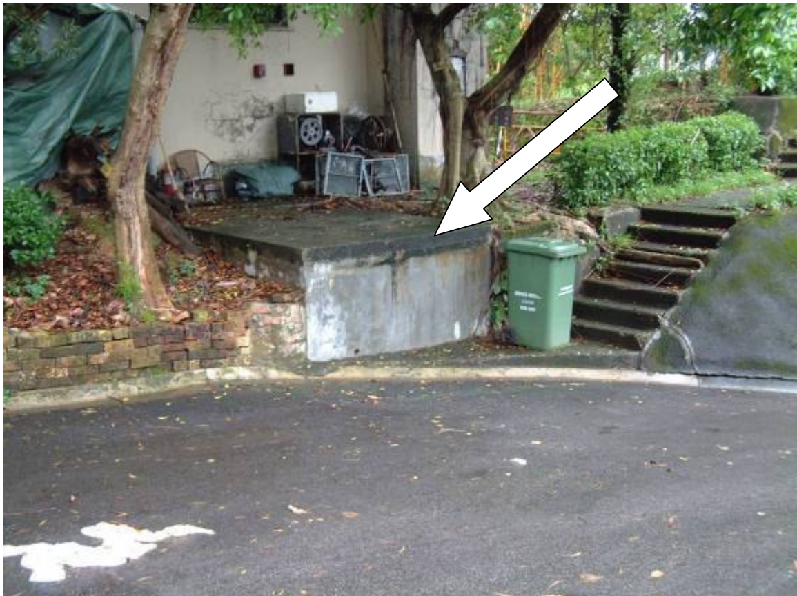
Photo 16 – Underground Fuel Tank in Skeletal Cremator Building
