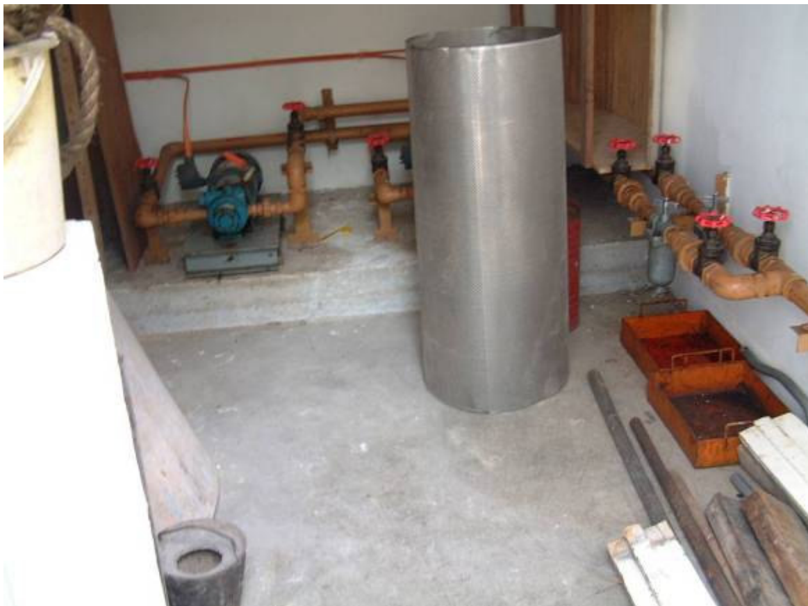
Photo 12 – Fuel Pump Room
