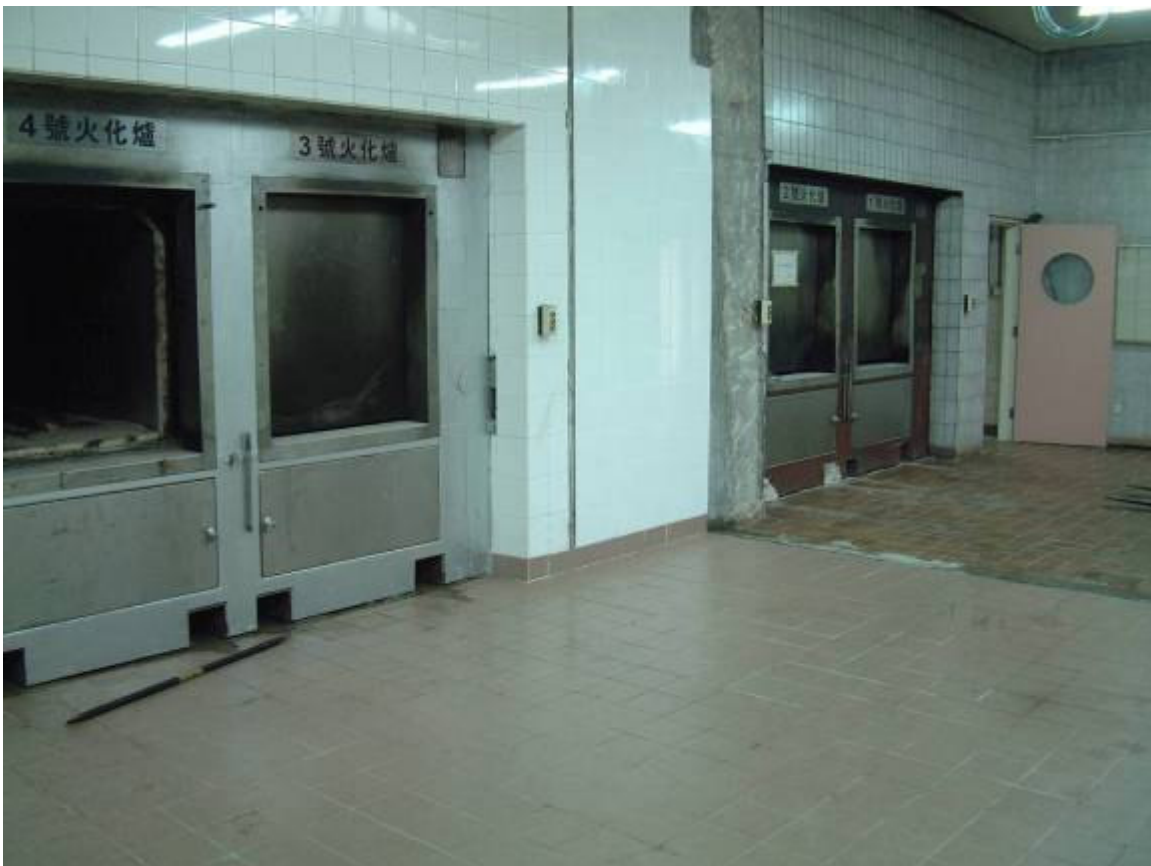
Photo 6 – Interior of Coffin Crematorium
